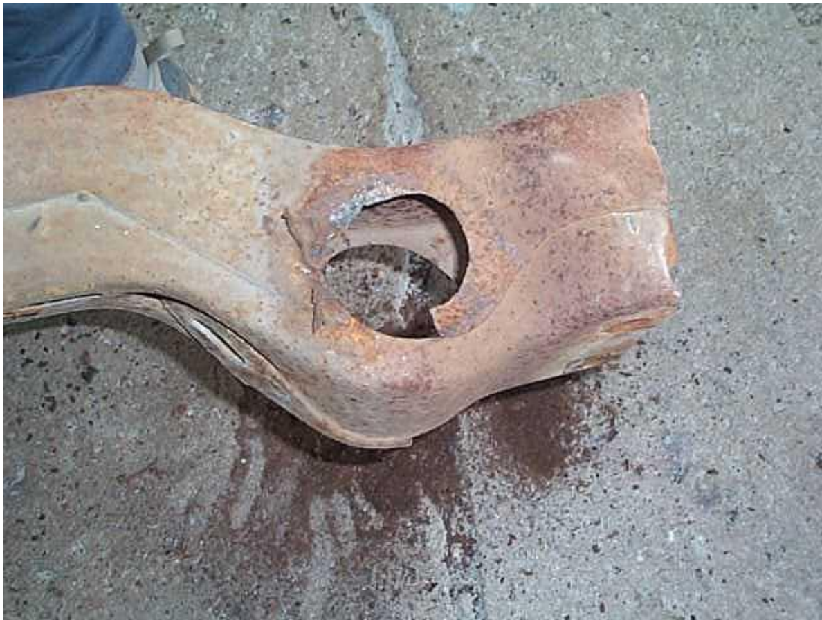
Body mount hole needing repair
